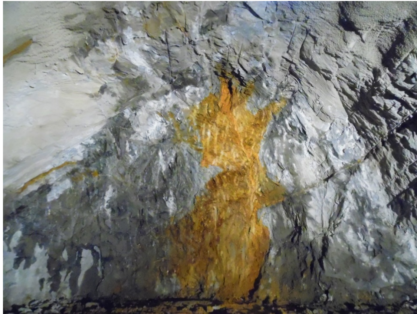
Figure 3 - Excavation face of Marão Tunnel (N Portugal) with a contact (by fault) between grey schists and quartzites
