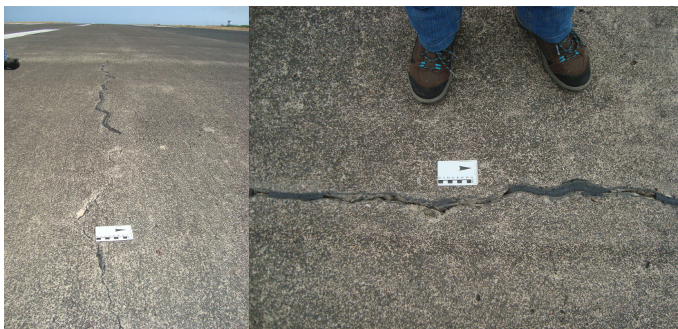
Fig. 1 – Image of the longest longitudinal crack pattern in the airport concrete pavement: (a) view N-S (left) and (b) a close-up of the crack (right).
