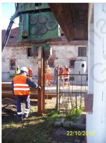
Fig. 1. Vibratory driving
