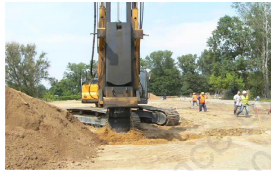
Fig. 5. Rapid Impulse Compaction
