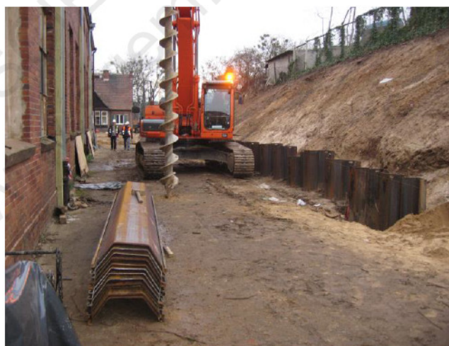
Fig. 2. Pre-boring before vibratory driving
